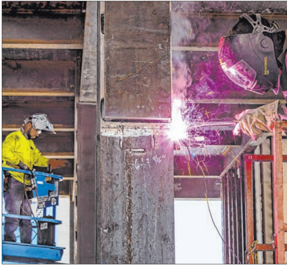
L.E. Baskow Las Vegas Review-Journal @Left_Eye_Images Jay Madrid, right, and Leonardo Mejia work on metal support beams Monday as construction continues on the multi-use commercial property in downtown Las Vegas.
